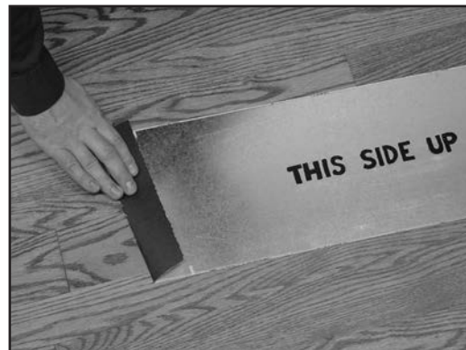
14. Locate notch and fold to notch.
